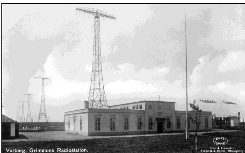
Varberg, Grimetons Radiostation.
